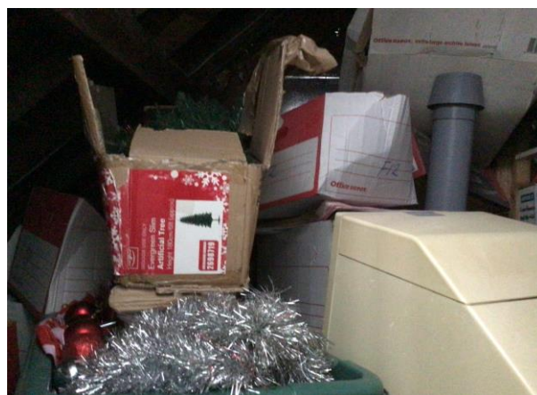
Combustible materials in loft area – main office
