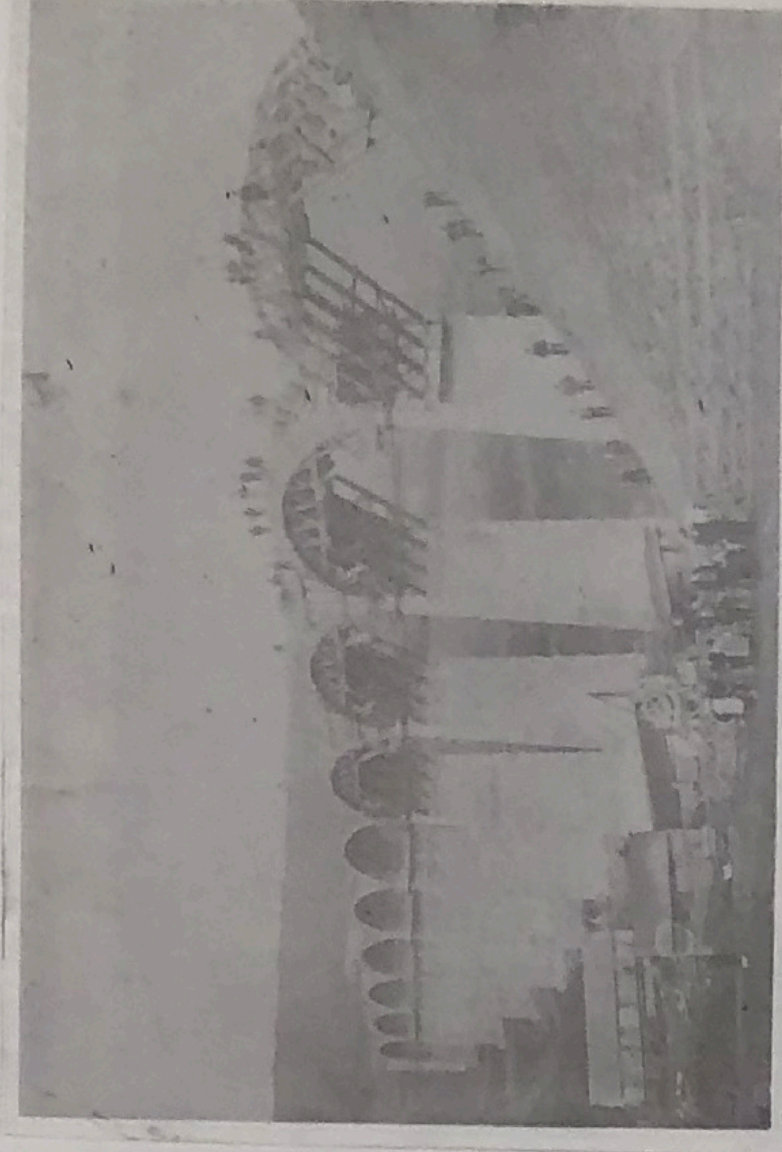
Camington Viaduct under construction, c. 1902. Constructed of concrete, this bridge on the Axminster to Lyne Regis railway is supported by nine piers. Note the 1,000 ft long cableway which spanned the valley and greatly assisted the workmen.
