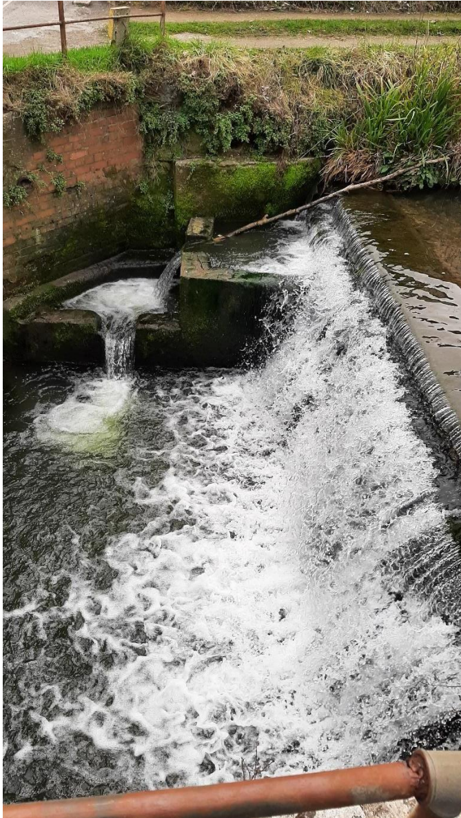
Figure 12 Fish pass weir
