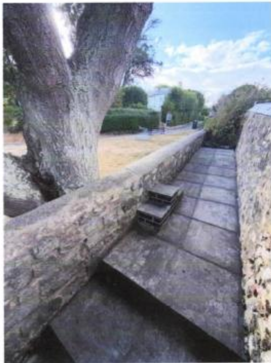
Step from alleyway to Langmoor Gardens over dwarf wall
