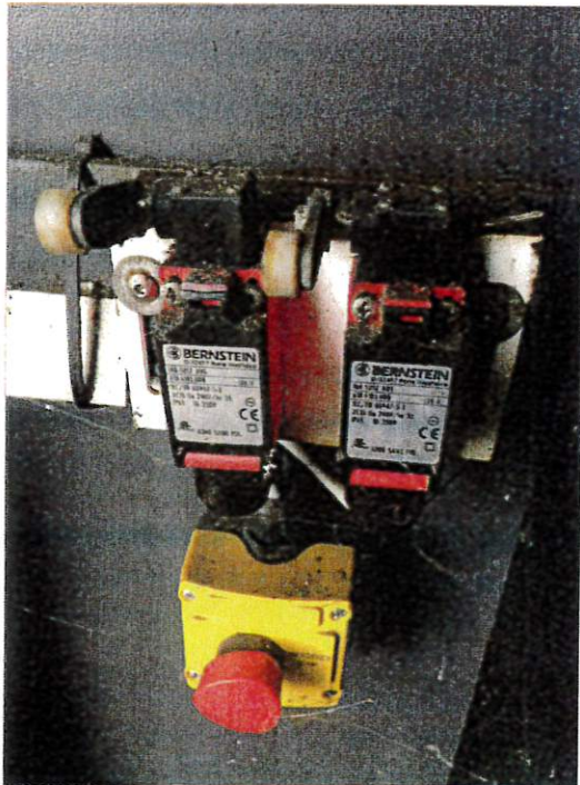
14 - Shaft switches need replacing
