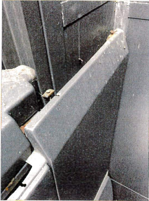
13 - Corrosion on screws and fixing
